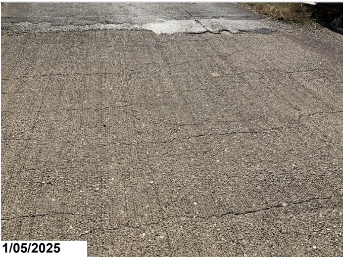
The topside of the deck has excessive amounts of cracking in various locations.
