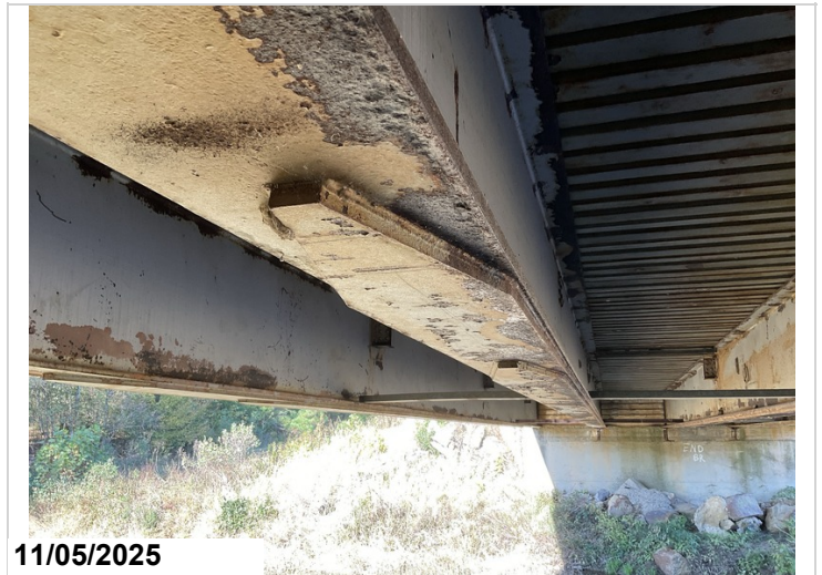
Cover plates are welded to the bottom flanges.
