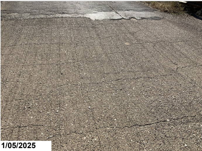
The topside of the deck has cracking in various locations, CS2
