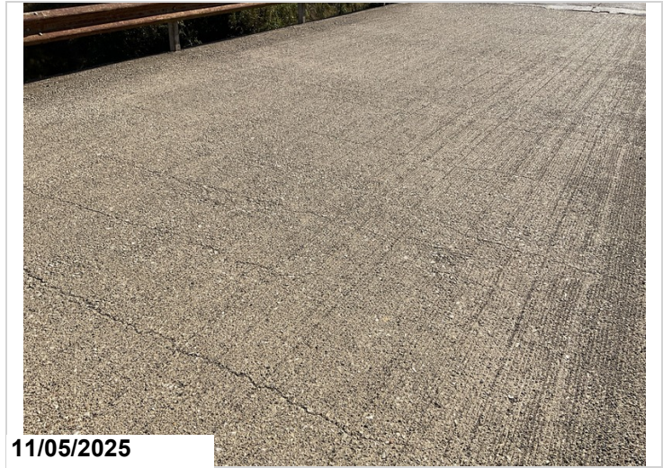
The topside of the deck has cracking in various locations, CS2
