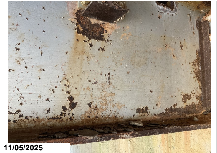
All steel beams have widespread minor corrosion in various locations, CS2.
